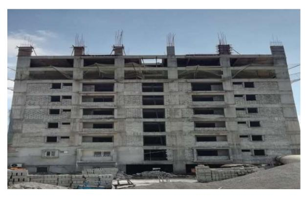
Block B2: Third Floor Level slab concrete casting 100% completed. Bar bending works for Columns up to fourth floor level on progress.
