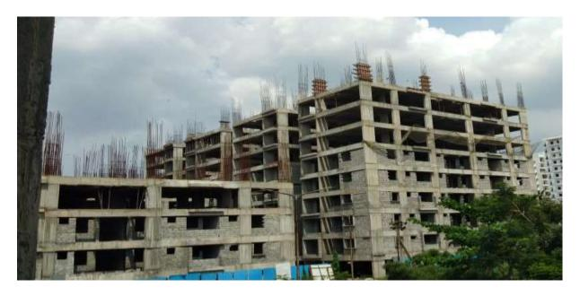
Block D3: Seventh Floor level slab First half concrete casting 100% completed. Barbending work for Second half of Seventh floor level on progress.
