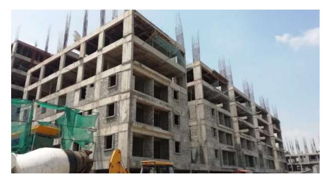
Block D1: Fourth Floor level slab First half concrete 100% completed. Shuttering & Barbending works for Second half of Fourth Floor level slab 75% completed.
