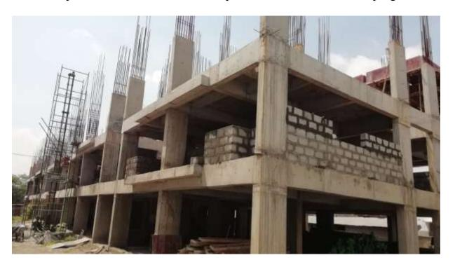
Block B1: Ninth Floor Level slab Concrete casting 100% completed. Column concrete upto Tenth floor level 35% completed and balance work on progress.
