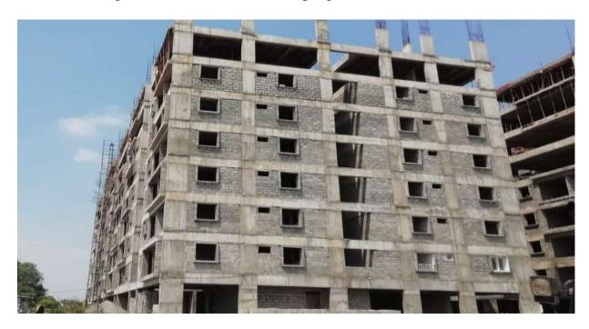
Block C2: Columns upto Ninth floor level 80% completed and balance works on progress. Slab Shuttering works at First half of Ninth Floor level 25% completed.
