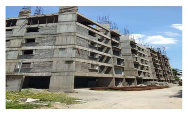
Community Hall: Third Floor level slab concrete casting 100% completed. Column concrete upto Fourth floor level completed.
